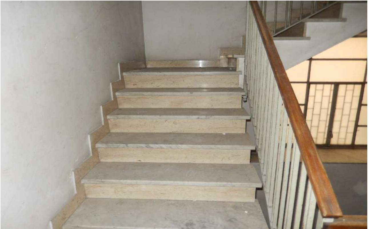
FO L1-11: scala condominiale;
